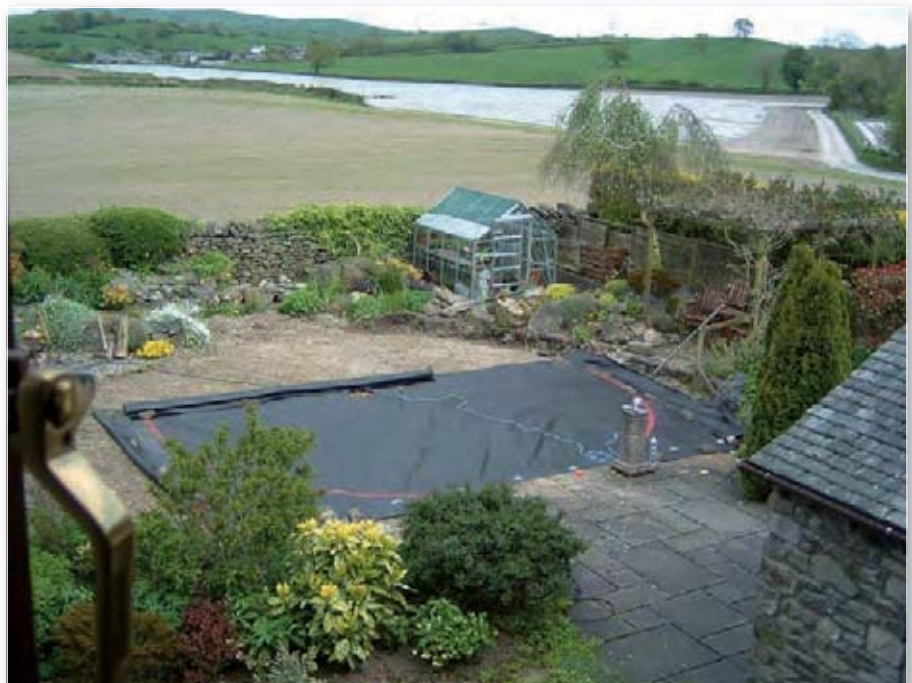
Fig. 13: Roy GOTAK laid a membrane (to protect the cables from corrosion) in the area, which was also filled with hardcore.
