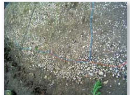
Fig. 12: Some of the radials had to be bent over to be accommodated in the available space.
